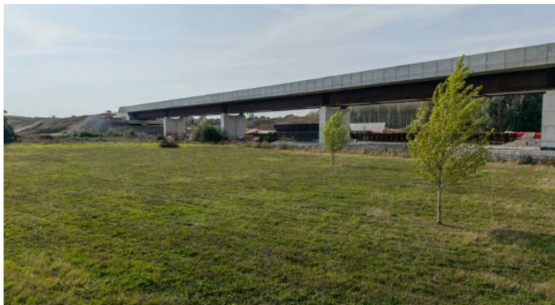
Pictured: Westbury viaduct
