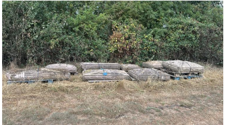
Pictured: Coping stones delivered
