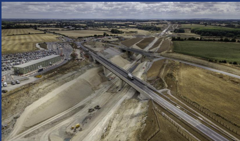
Pictured: The A422 overbridge opened to traffic
