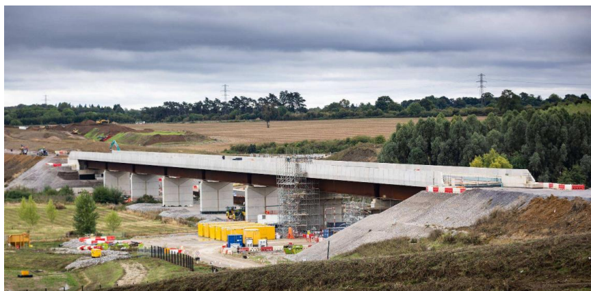
Pictured in July 2026: A view of Westbury viaduct, which was structurally completed in September 2026
