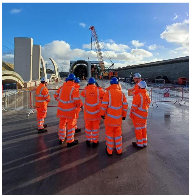
Pictured: A site visit with a local group at the Wendover green tunnel
