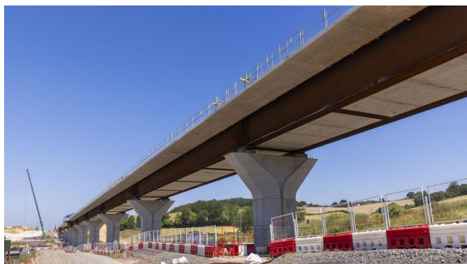
Pictured: Wendover Dean viaduct following top deck concrete pour completion
