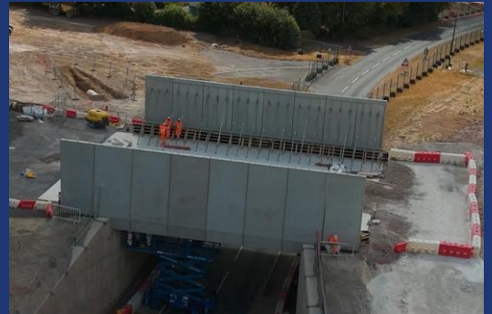
Pictured: Parapets installed on the Rocky Lane underbridge. View the progress video below:
