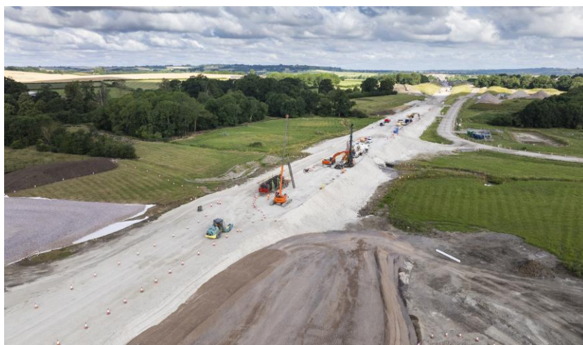
Pictured: The Oxford Road embankment between Hartwell and Coldharbour, showing piling works in preparation for the acoustic barrier and the site of the future SBH/32 footbridge (July 2026)
