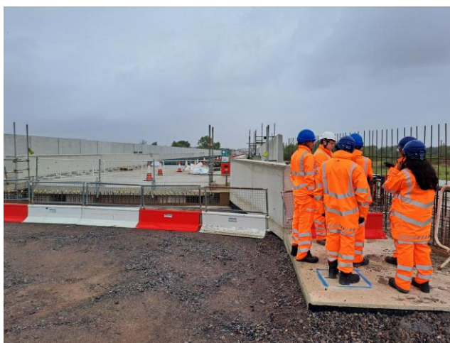
Pictured: A recent site visit with a local group to Thame Valley Viaduct near Aylesbury
