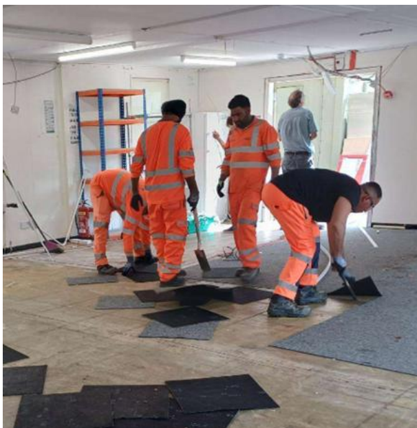
Pictured: Teams helped remove the old floor of the food larder ahead of renovation works.
