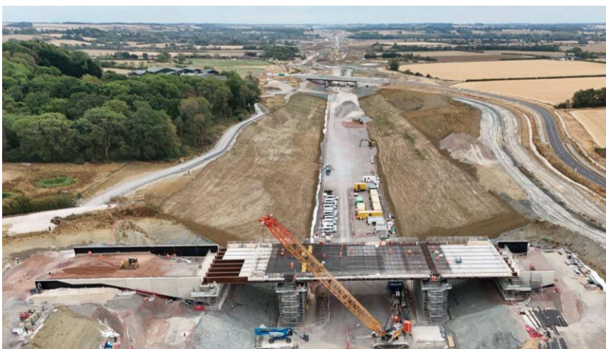
Pictured: The deck structure is being completed, and parapets will be installed this autumn at Stoneton Lane green overbridge.
