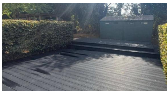
Pictured: Constructing a frame and laying durable decking and painting the storage shed has transformed this area for the children.
