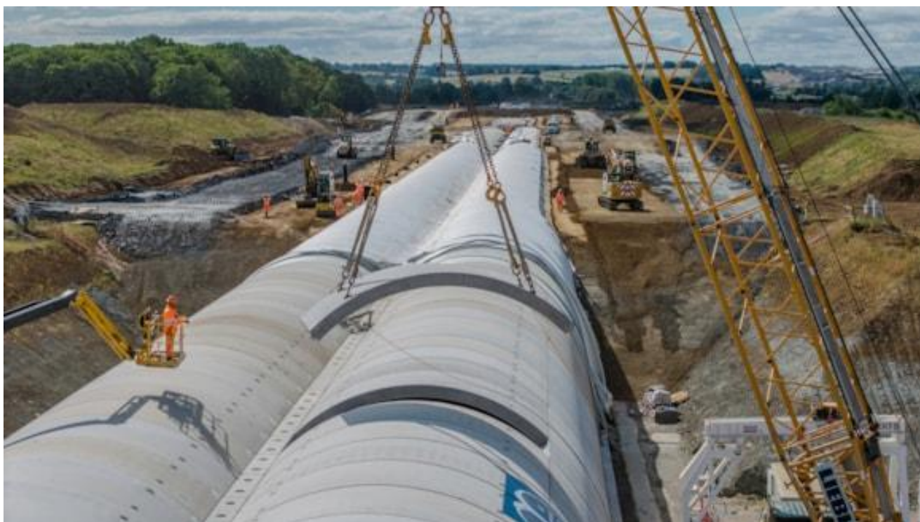
Pictured: The final reinforced concrete section is installed at the Chipping Warden green tunnel.
