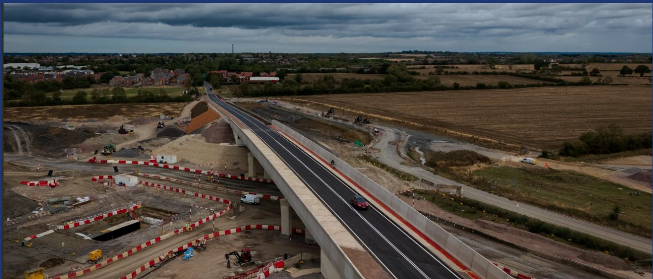
Pictured: A423 road bridge opens near Southam.
