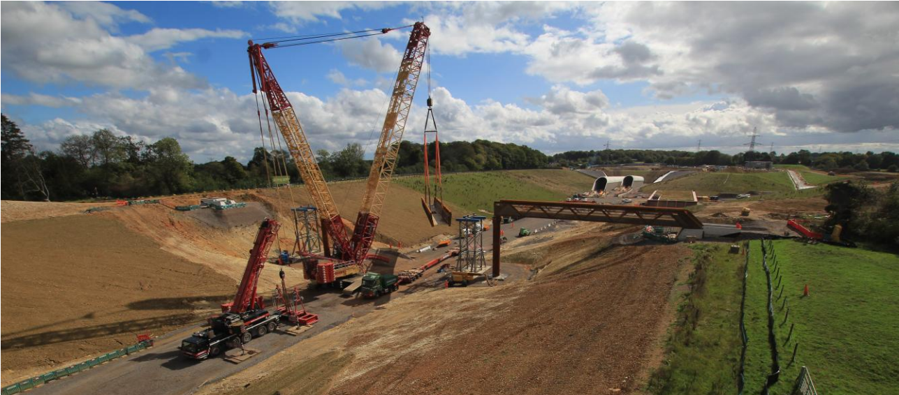
Above: Deck sections for GMI/12 being installed across the cutting in September 2026.
