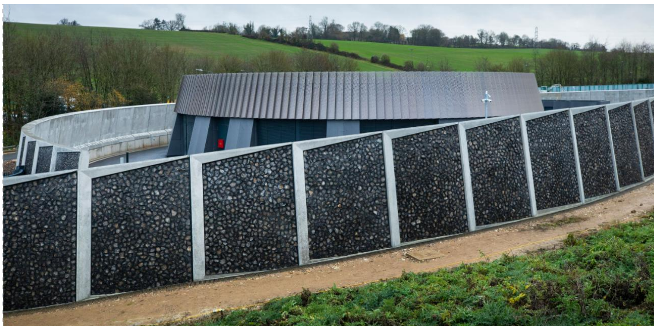
Above: Amersham ventilation shaft building pictured from the site boundary.
