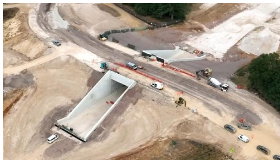
Above: Leather Lane bridge construction in August.
