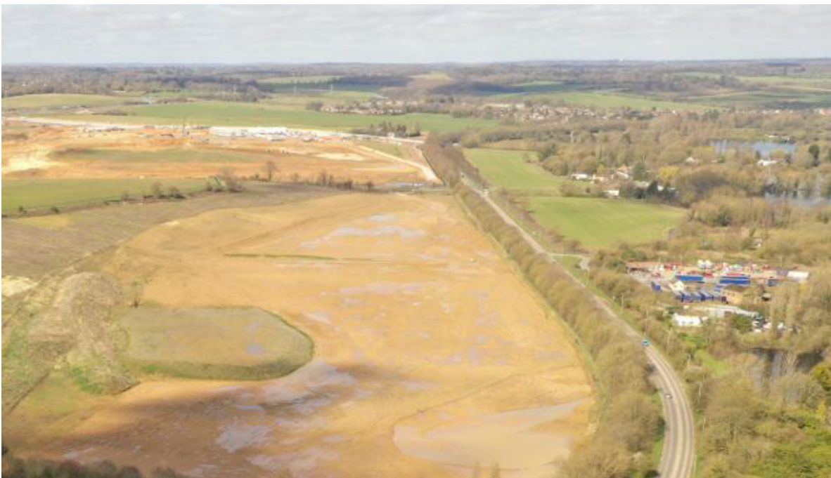
The same viewpoint of the site at the start of Align's works in March 2020.
