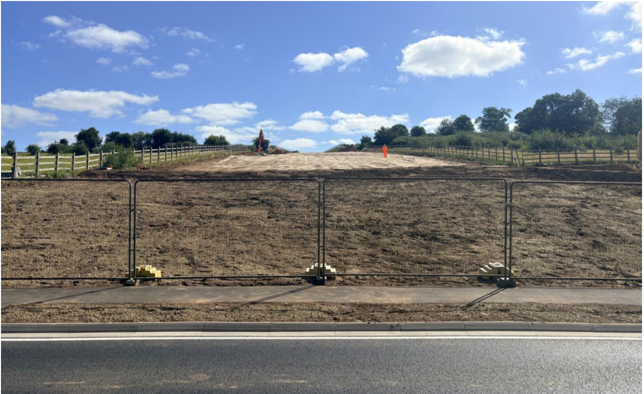
The A413 Amersham Road following the removal of the temporary access road near Chalfont St Peter in late June 2026.
