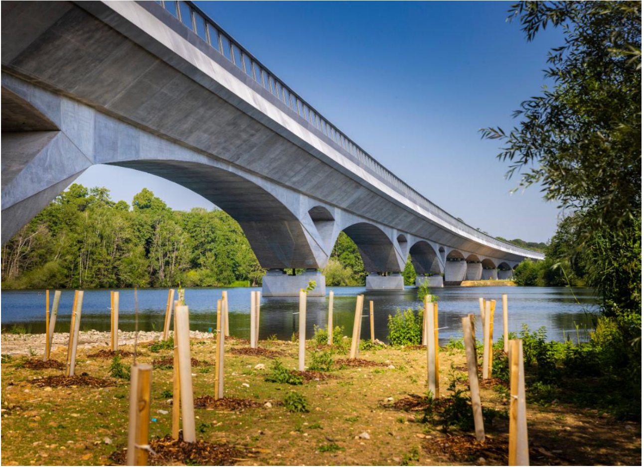
Lakeside planting along the route of the Colne Valley viaduct.
