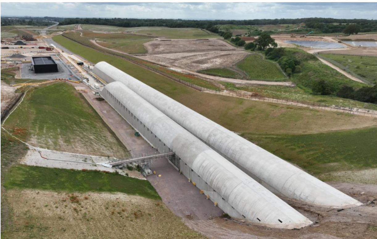
The Chiltern tunnel south portal nestled in the calcareous grassland near Maple Cross, Hertfordshire.
