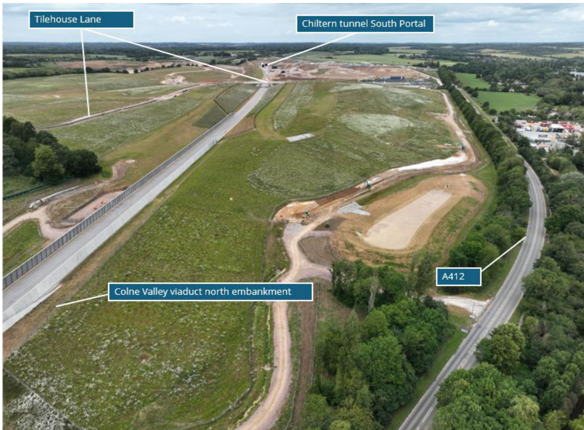
The Chiltern tunnel south portal site (top of frame) and the approach to the Colne Valley viaduct, June 2026 including permanent pond and planting on chalk placement.
