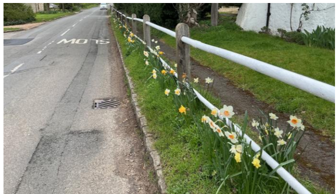
Water Stratford railings.
