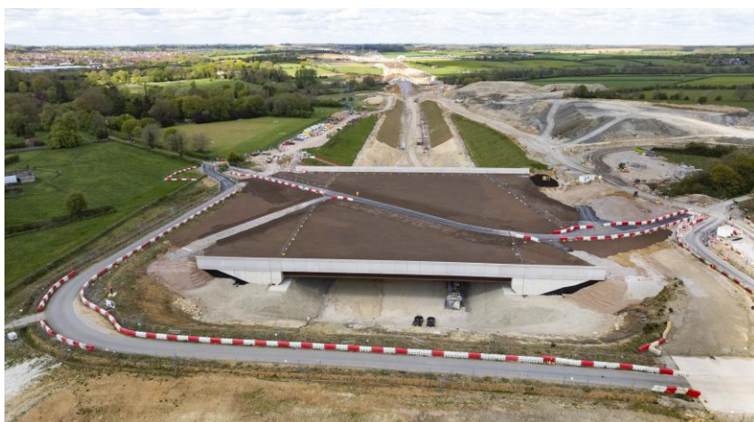
Pictured: Turweston Green overbridge
