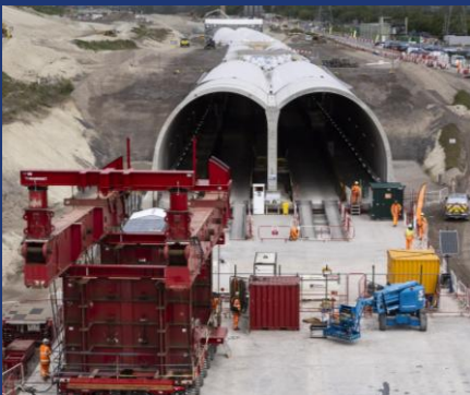
Pictured: SPMT working at the Wendover green tunnel
