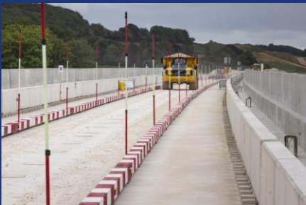
Pictured: Small Dean viaduct in use as a mass haul route for our construction vehicles
