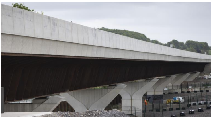
Parapets installed across the Small Dean viaduct in April 2026
