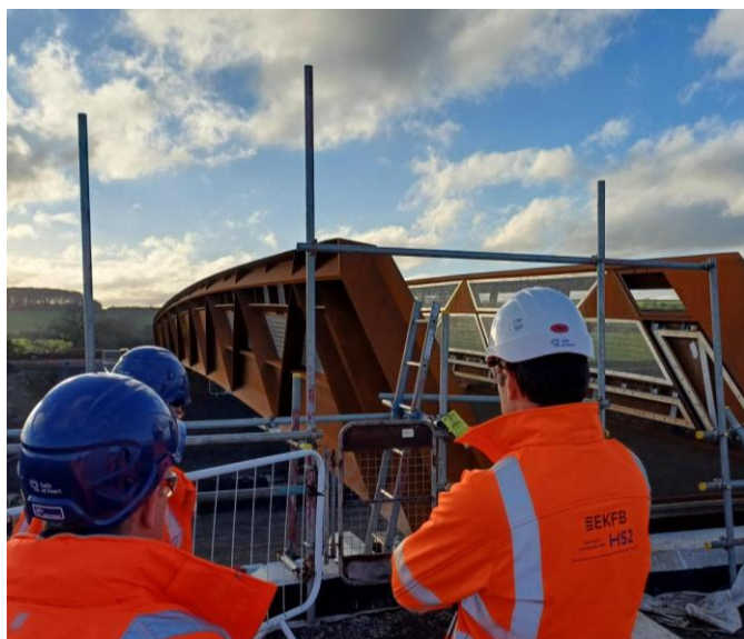
Pictured: A recent site visit with a local group to the Greenway footbridge near Waddesdon, which is due to be open this autumn
