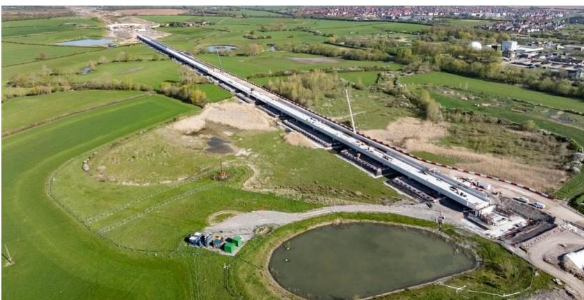
Pictured: The 880-metre-long Thame Valley Viaduct, showing construction progress, with its concrete base completed and side walls (parapets) installed May 2026
