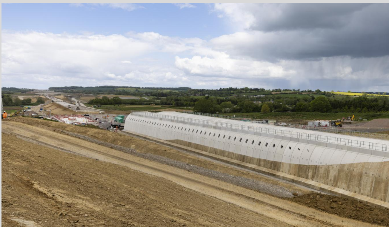
Pictured: Progress continues at the Chipping Warden green tunnel, with the waterproofing layer now visible on the portal, showing how the tunnel will emerge from the ground as backfilling works carry on this year.
