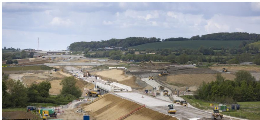
Pictured: View looking North from Chipping Warden green tunnel towards Highfurlong Brook viaduct and three road bridges crossing the HS2 railway line.
