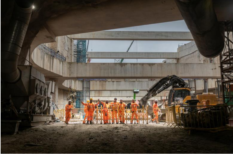
Inside the Victoria Road Crossover Box
