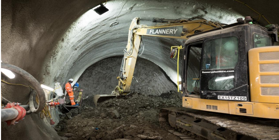
Step 1: Excavation of a tunnel using an excavator
