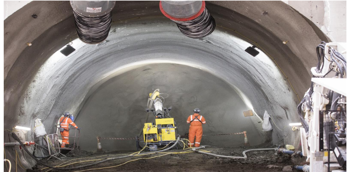
Step 2: Application of primary sprayed concrete.
