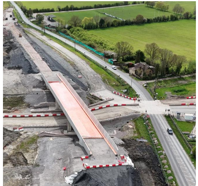
Earthworks for the Kineton Road bridge approach roads are built to join the bridge to the local highway network.
