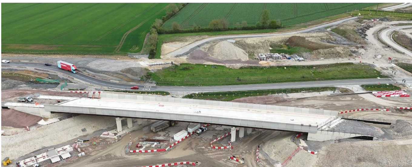
The HS2 railway line will pass under the A423 road bridge, currently under construction.
