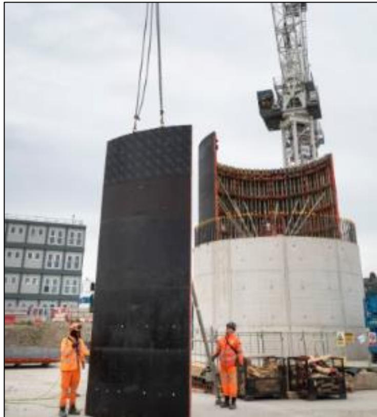
Progress of ventilation column construction
