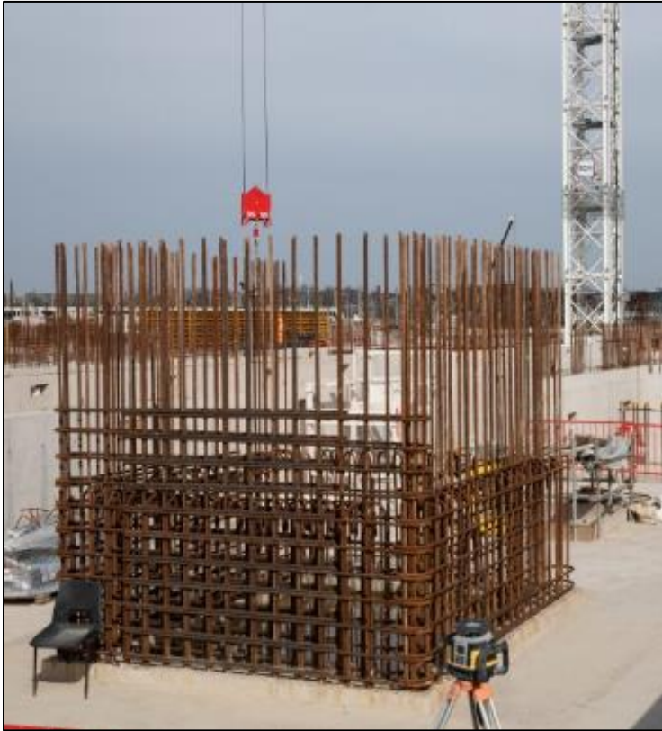
Platform lift shaft & external invert walls
