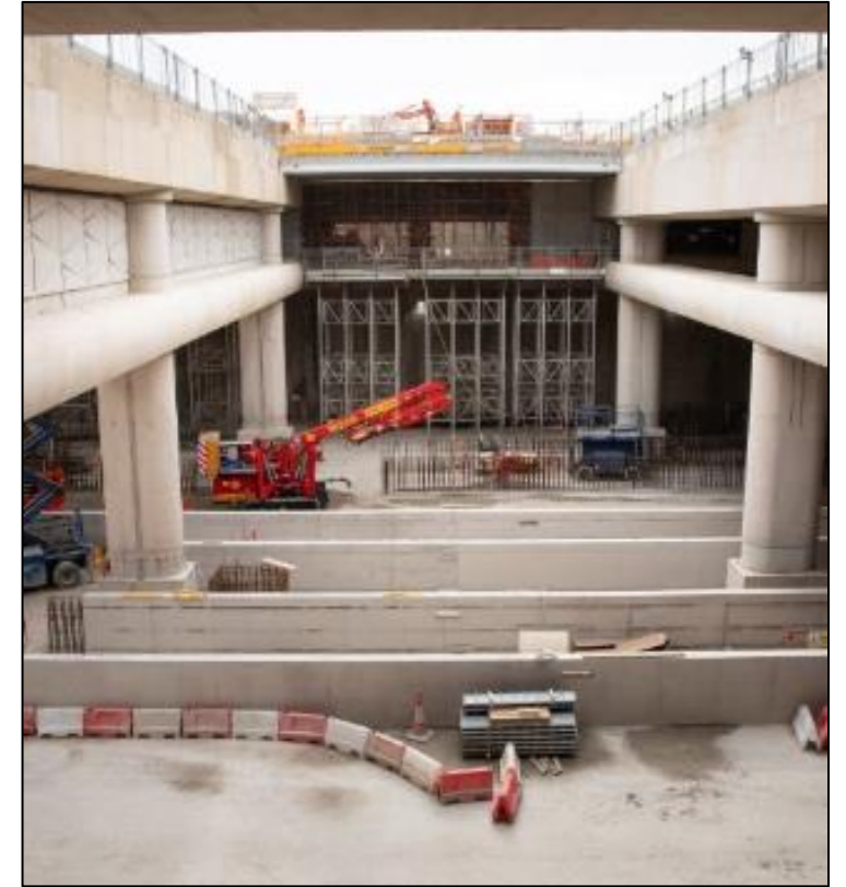
Smokedown stand and platform walls
