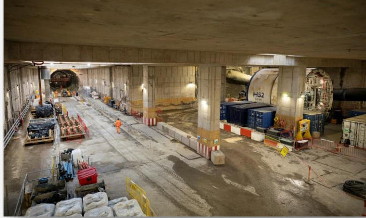
View from within the East Box at Station site
