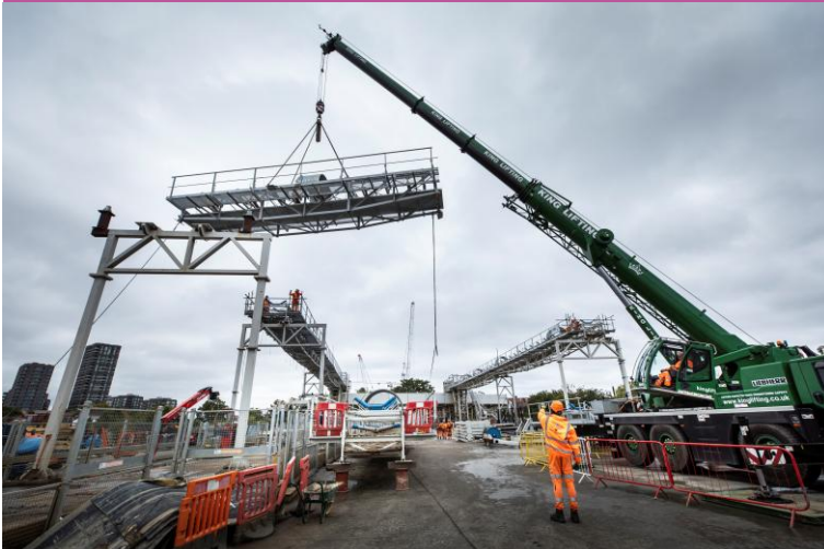
Removal of conveyor system in Flat Iron site
