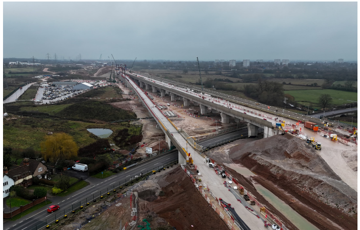
Coleshill viaducts crossing the B4114
