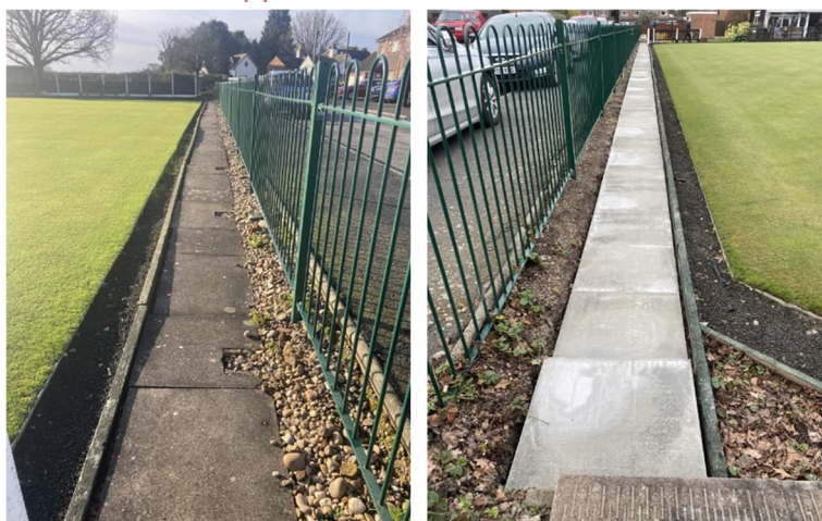
Water Orton Bowls Club – removing and replacing old slabbing
