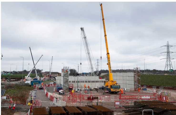
M42 Motorway twin box
