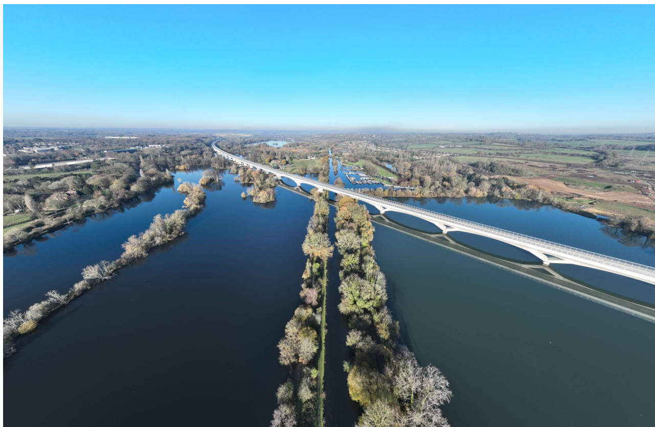
A view of the completed Colne Valley viaduct looking from Hillingdon towards Buckinghamshire and Hertfordshire.
