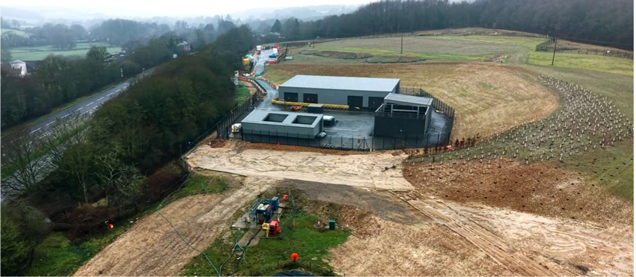
Little Missenden ventilation shaft site.
