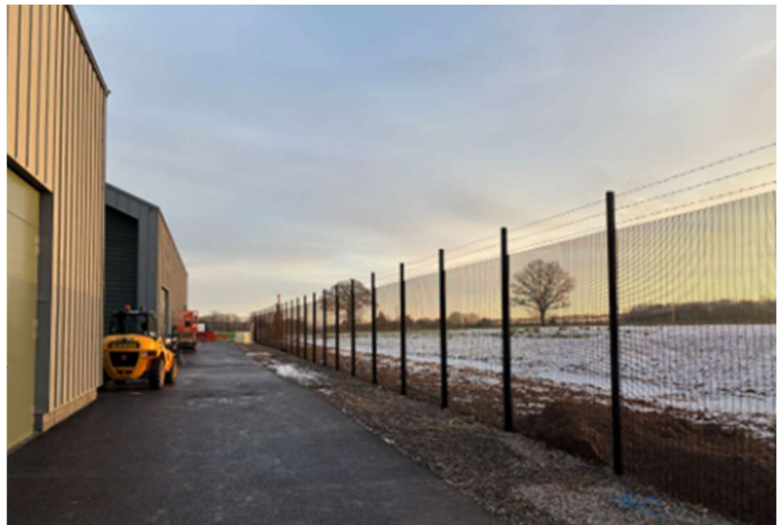
Chesham Road ventilation shaft buildings.
