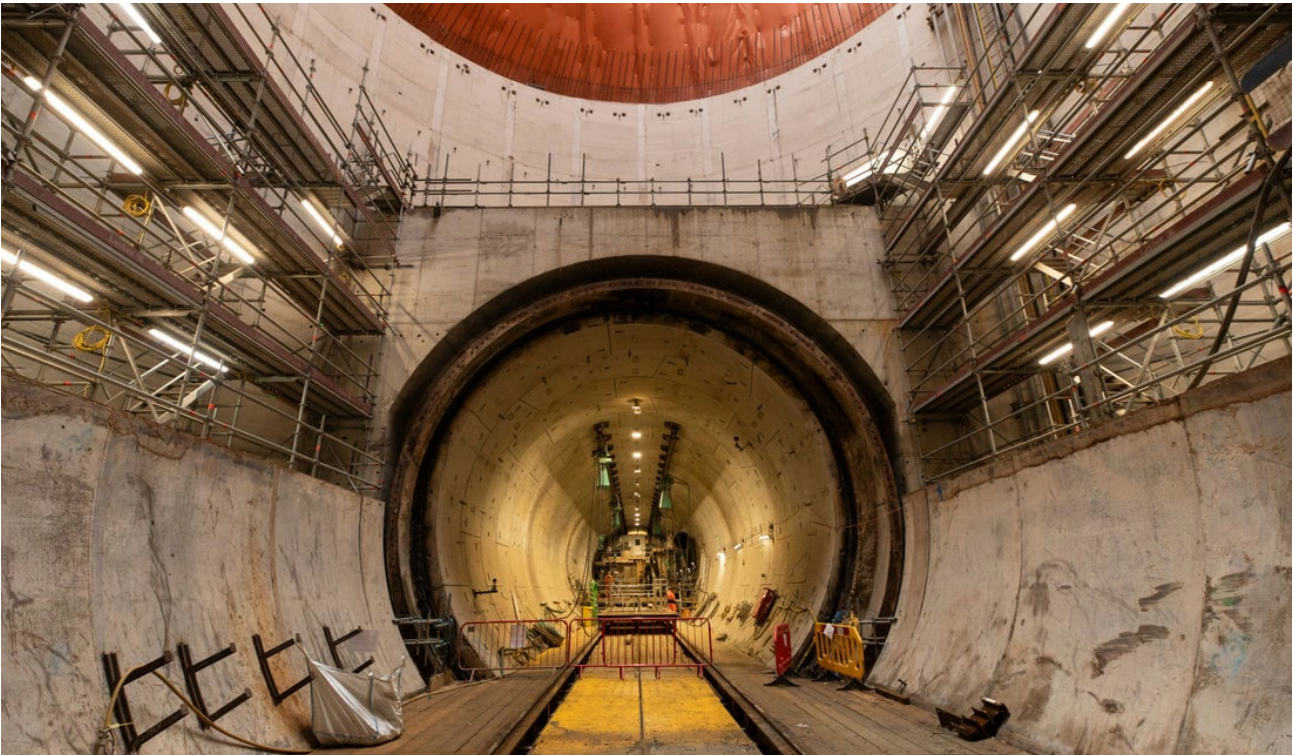
Inside one of the Northolt tunnels
