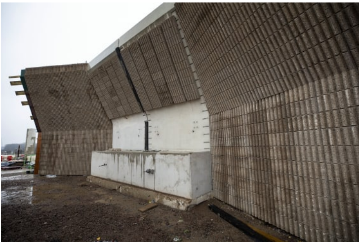
Images showing the piling and first concrete panels for the noise barriers
