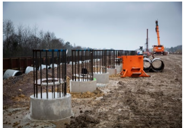
Images showing the piling and first concrete panels for the noise barriers
