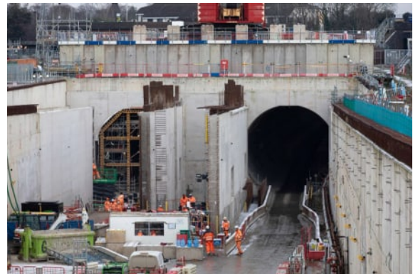
West Ruislip Tunnel portal
