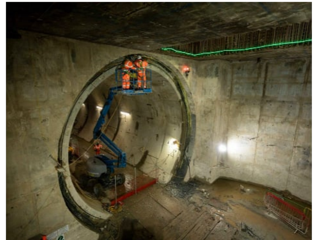
Mandeville Road vent shaft tunnel connection
