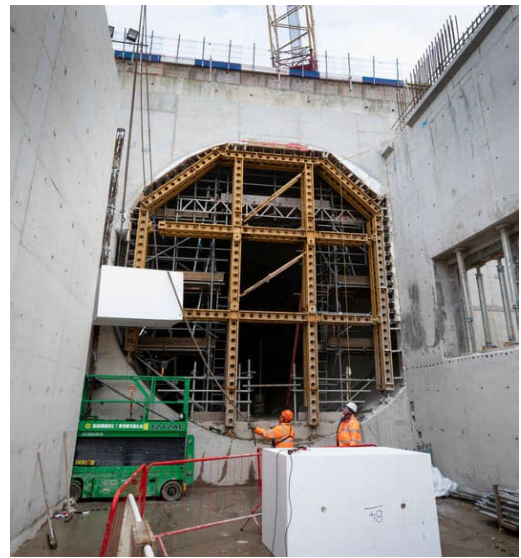
West Ruislip portal progress
