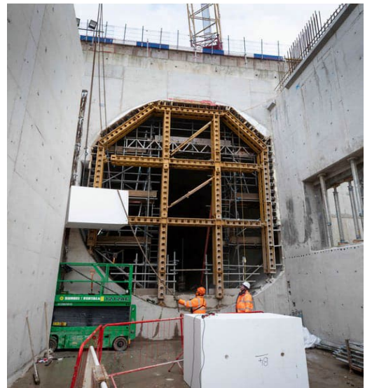
West Ruislip portal progress
