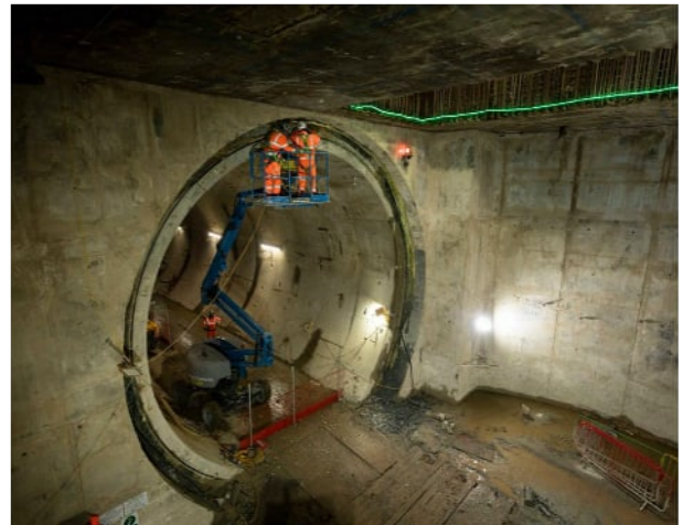
Mandeville Road vent shaft tunnel connection
