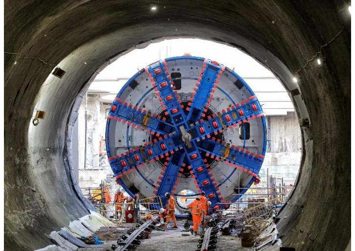
Above: TBM cutterhead
