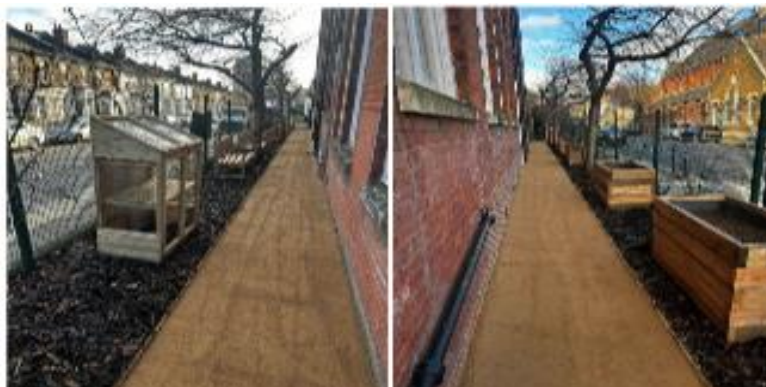
Above: Kenmont Primary School: Garden Renovation project
