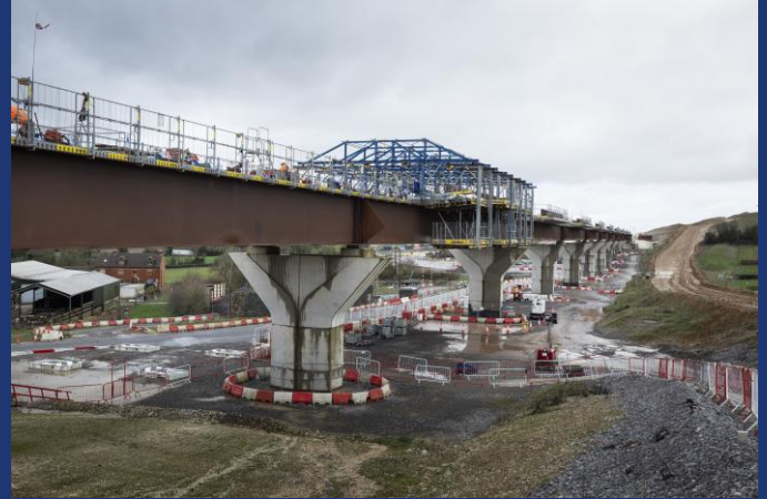
Wendover Dean viaduct, February 2026
