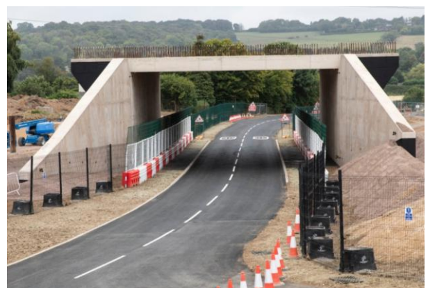
Rocky Lane underbridge and permanent realignment
