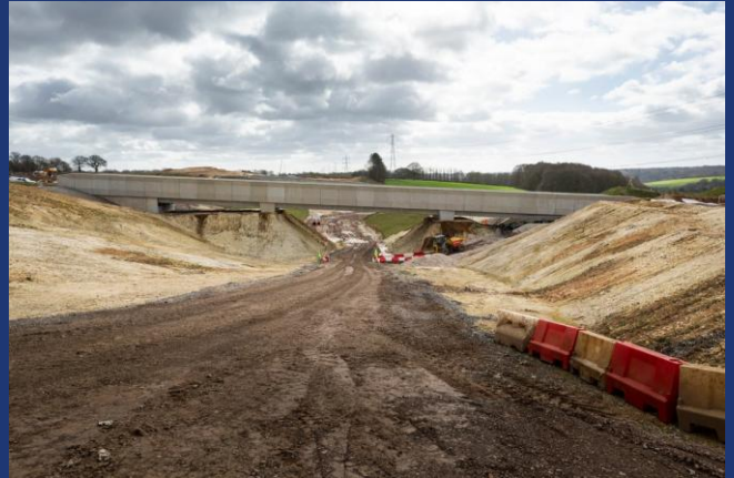
Bowood Lane overbridge, March 2026
