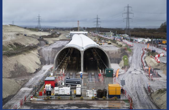
Wendover green tunnel construction, February 2026
