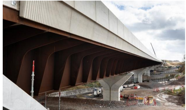
Small Dean viaduct, March 2026
