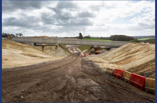
Bowood Lane overbridge, March 2026
