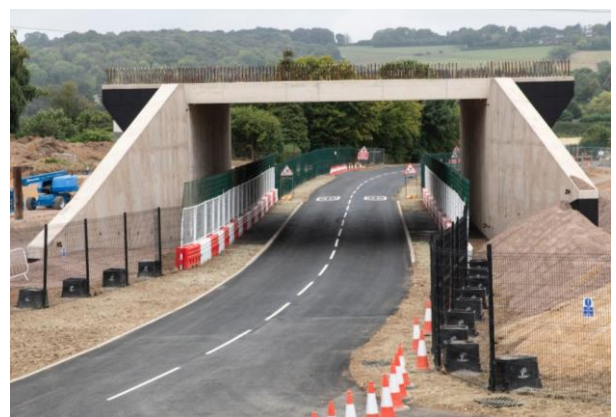
Rocky Lane underbridge and permanent realignment
