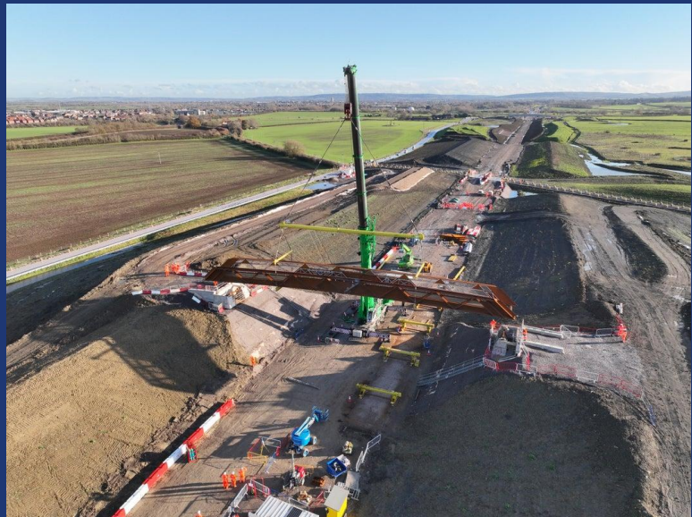
Right: The Waddesdon Greenway bridge deck lift in December 2025
