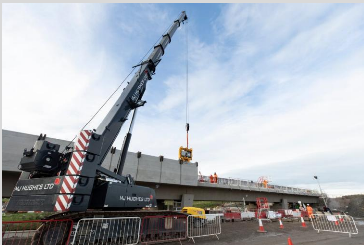
Left: pre-cast parapet sections being lifted into place using the suction frame
