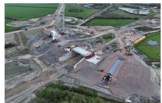
Network Rail overbridge top left, Station Road overbridge central and a cycle/pedestrian under path bottom right.
