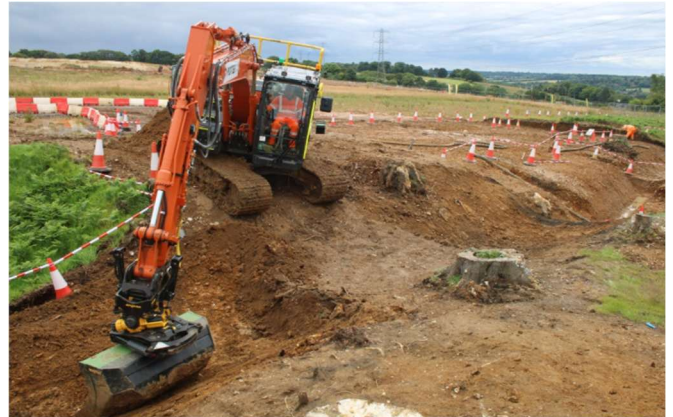
A 20T excavator creating a drainage channel in Buckinghamshire.
