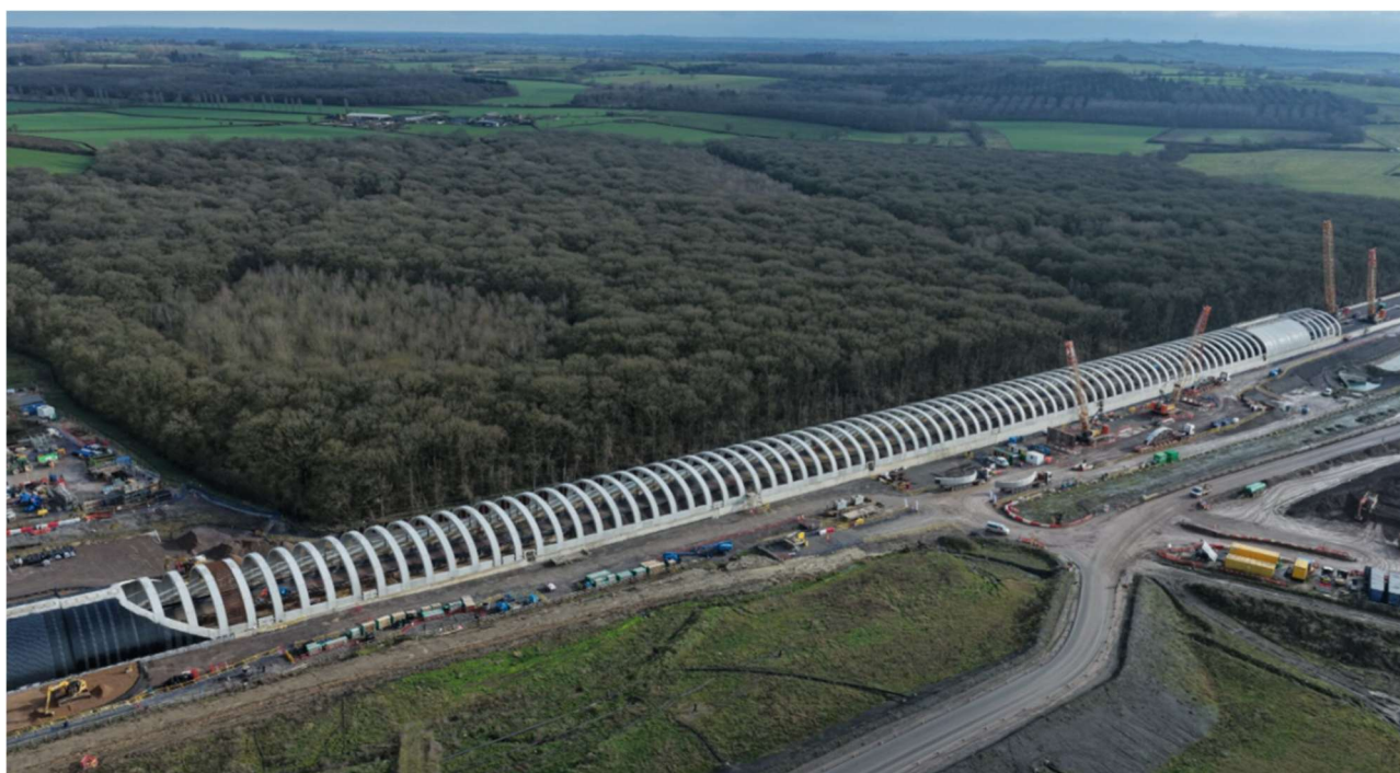
The image above shows Sheephouse Wood with the 1km bat protection structure spanning the woodland edge.
