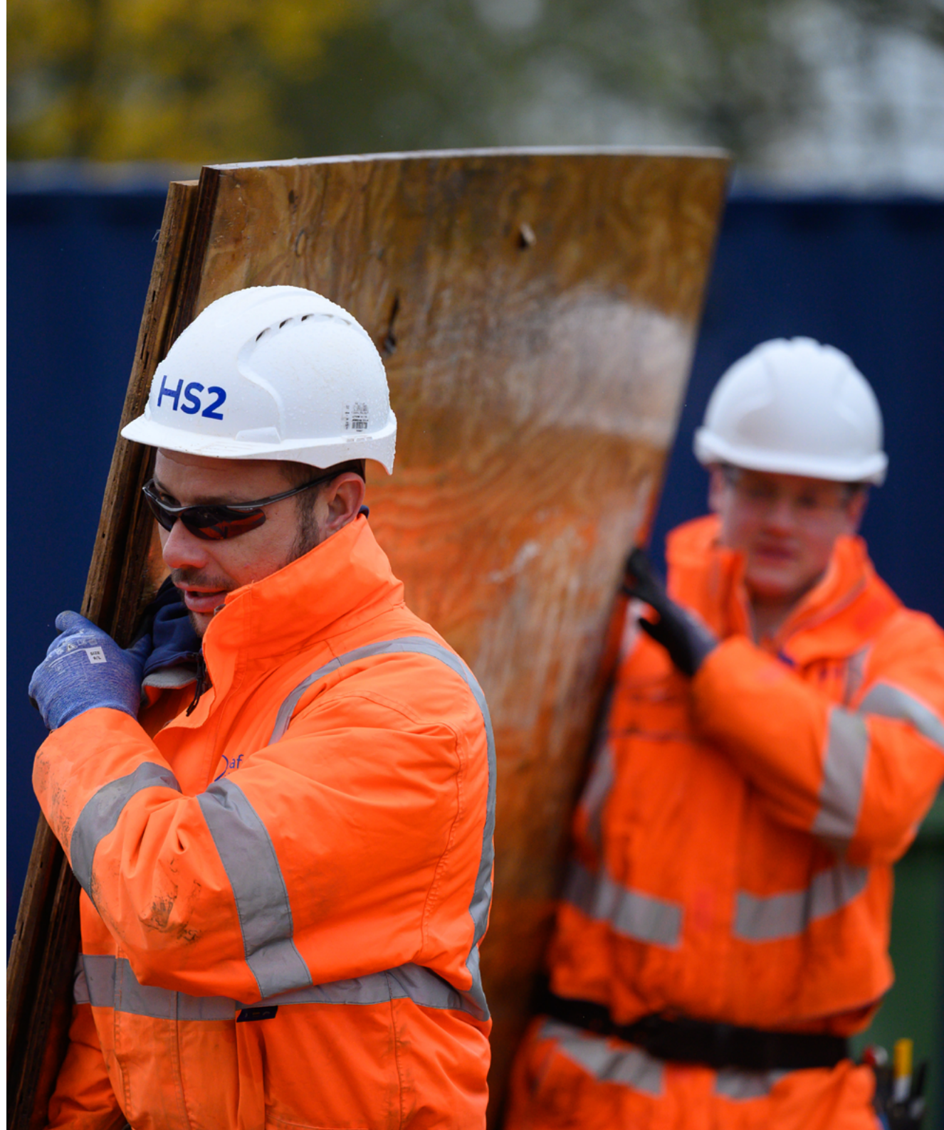
Image: Workers lifting equipment on site
