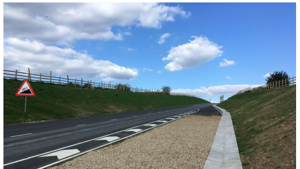
The temporary access road linking the Chalfont St Peter construction site to the A413 London Road will be removed this year.
