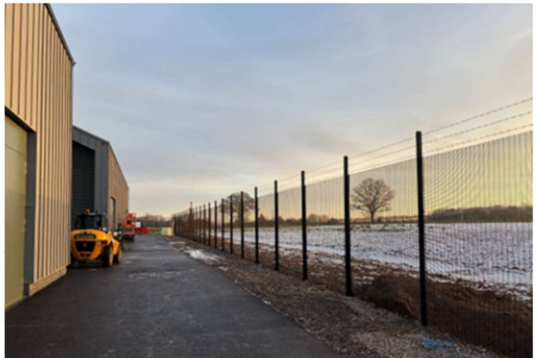
Chesham Road ventilation shaft buildings.
