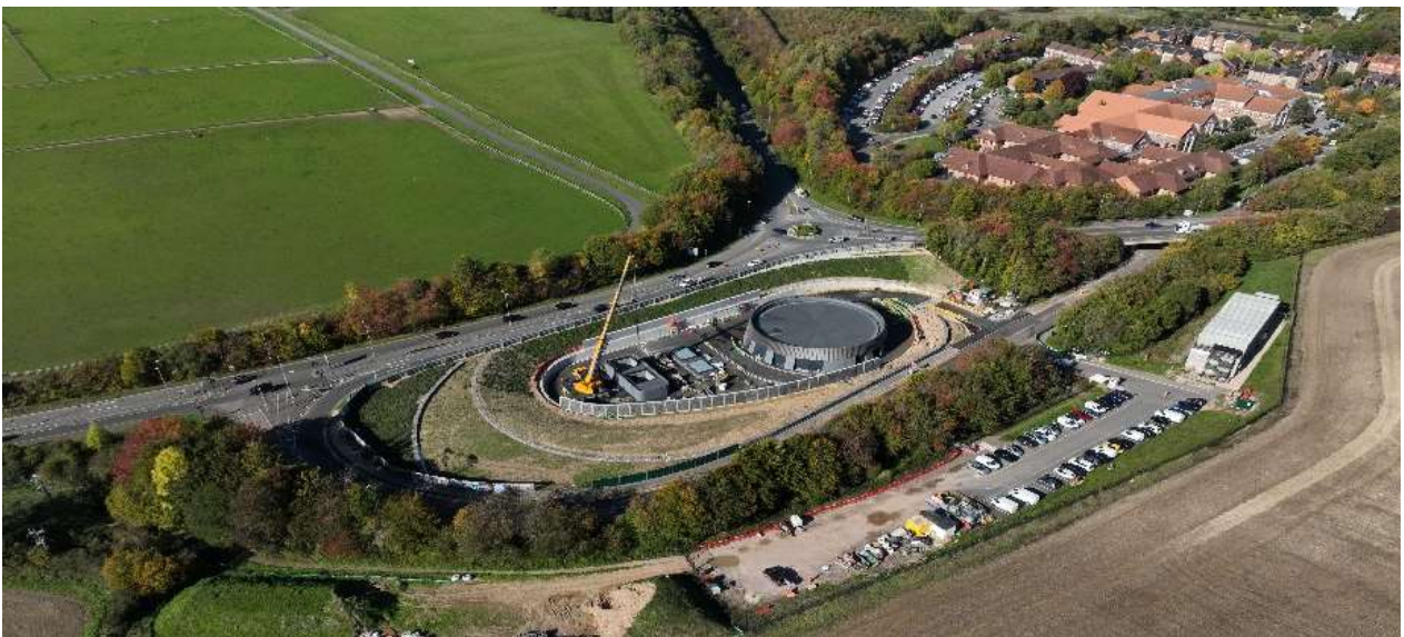
Amersham ventilation shaft as seen from the air.
