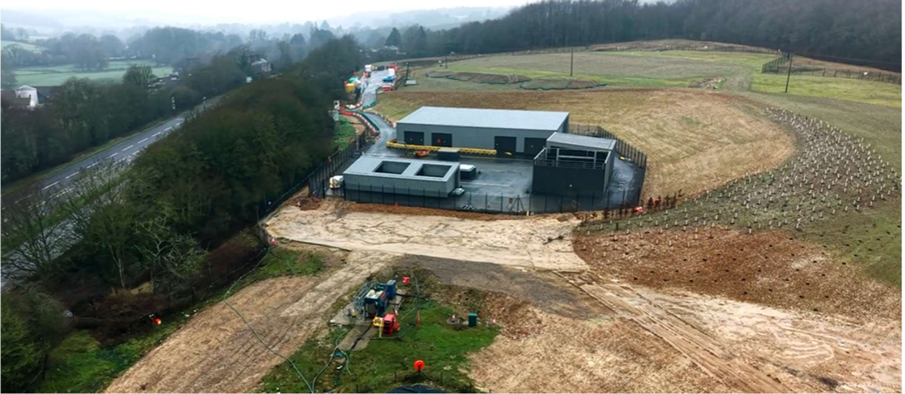
Little Missenden ventilation shaft site.
