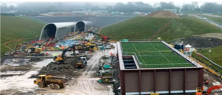
A view of the Chiltern tunnel north portal and ancillary building, looking toward Frith Hill, from February 2026.
