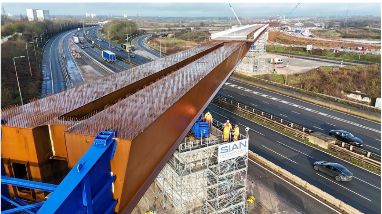
Image of the M6 South viaduct East Deck across the motorway.
