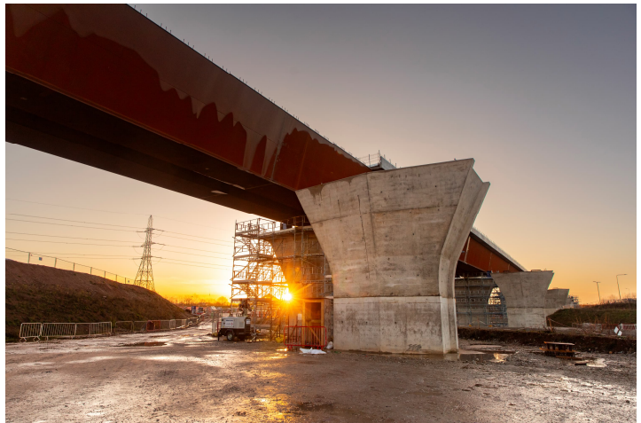
M6 South viaduct progress
