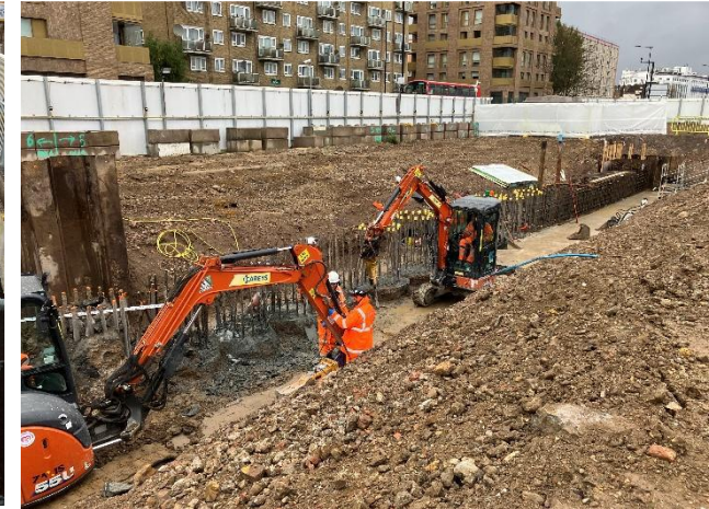
Retaining Wall and Piling
