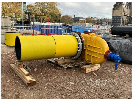
Image showing inserted gas valve on Drummond Street works (inside our site)
