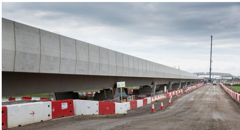
Left: The Thames Valley Viaduct with newly installed concrete parapets
