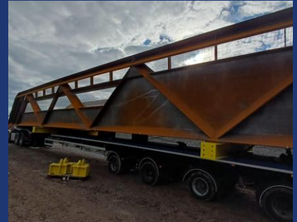
Above: a section of the new Greenway bridge
