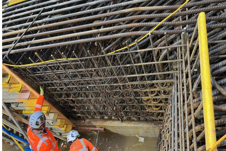
Reinforced concrete structure in satellite shaft
