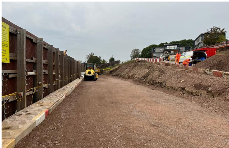
H pile platform for ground stabilisation
