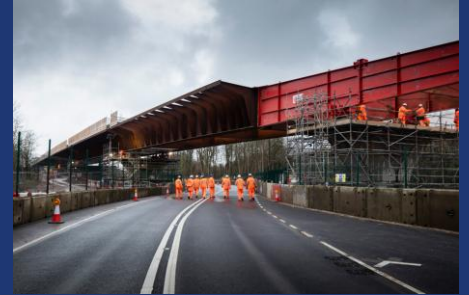
Small Dean viaduct, February 2025
