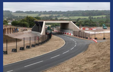
Rocky Lane realignment in operation
