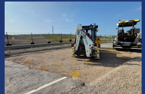
Reinstating Nash Lee Road following the closure in August 2025
