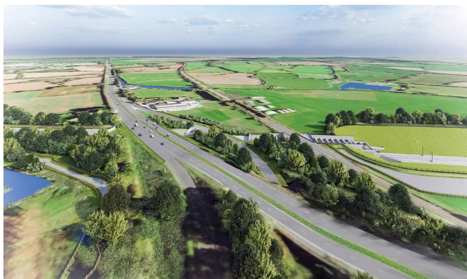
HS2 Streethay cutting under the A38
