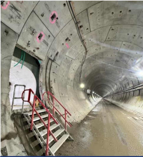
A completed cross passage in Northolt Tunnel
