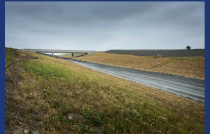
Above – A41 Overbridge at Waddesdon South Cutting
