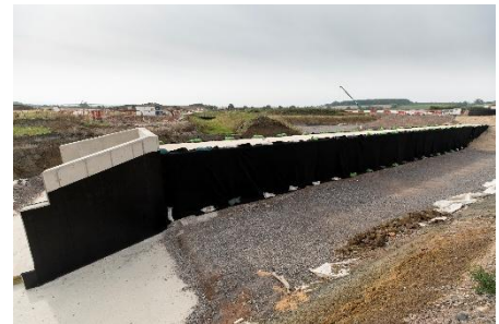
Above – waterproofing before backfilling, Fleet Marston Culvert
