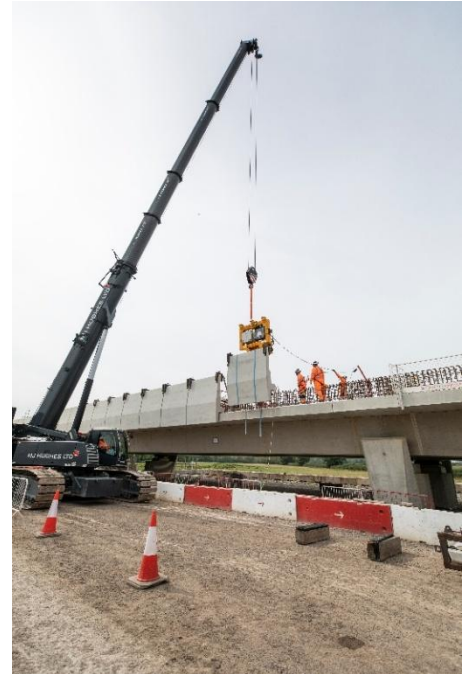
Above – Parapet section being lifted into place at the Thame Valley Viaduct
