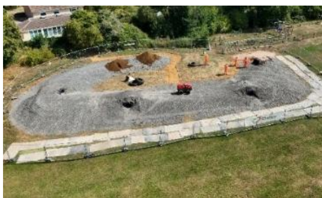
Running track during construction
