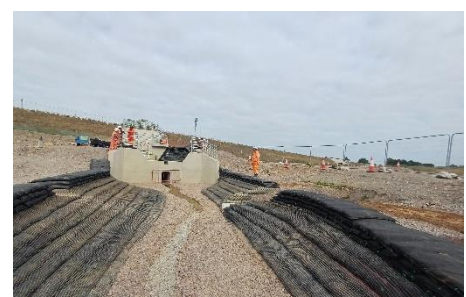
Above – Stoke Brook running through the new PRA culvert
