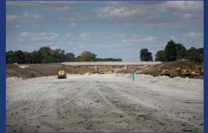
Above – Oxford Road Cutting towards A418 Overbridge
