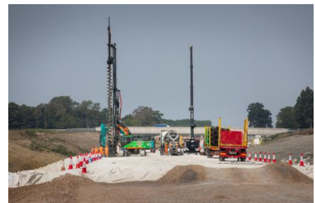
Above – Noise barrier piling rigs in use, Oxford Road Cutting
