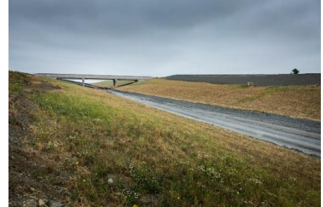
Above – topsoiling at Waddesdon South Cutting
