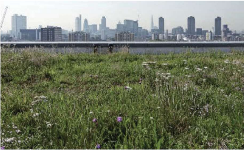
5. GREEN ROOF Intensive Green Roof with deep growing substrate and biodiverse planting of grasses, herbaceous and shrub planting.
