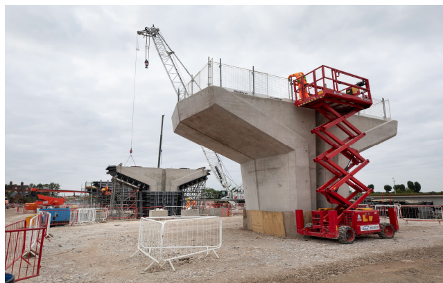
River Blythe Viaduct pier construction and groundworks
