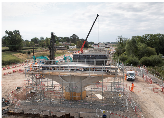
Visual showing construction progress of Balsall Common Viaduct
