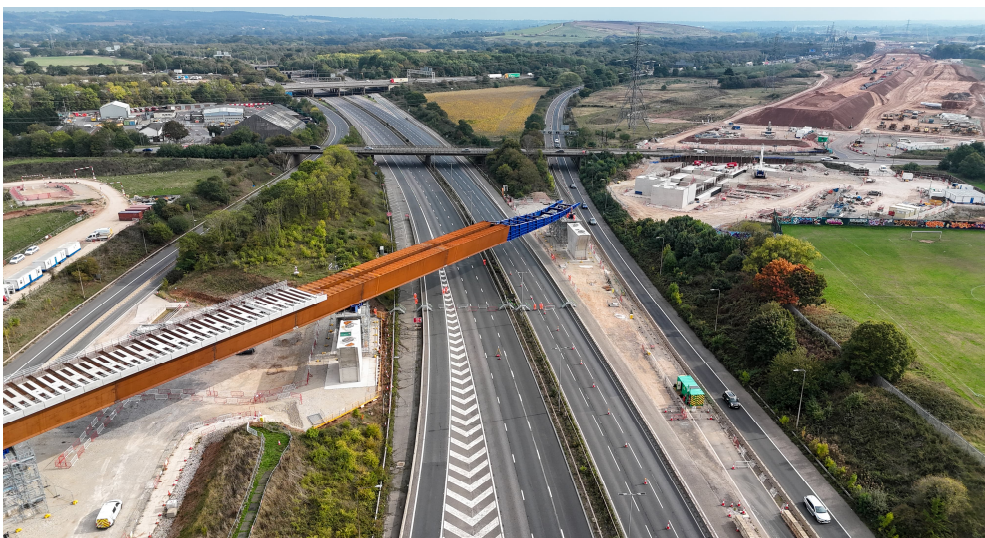
M6 South viaduct East Deck over the motorway
