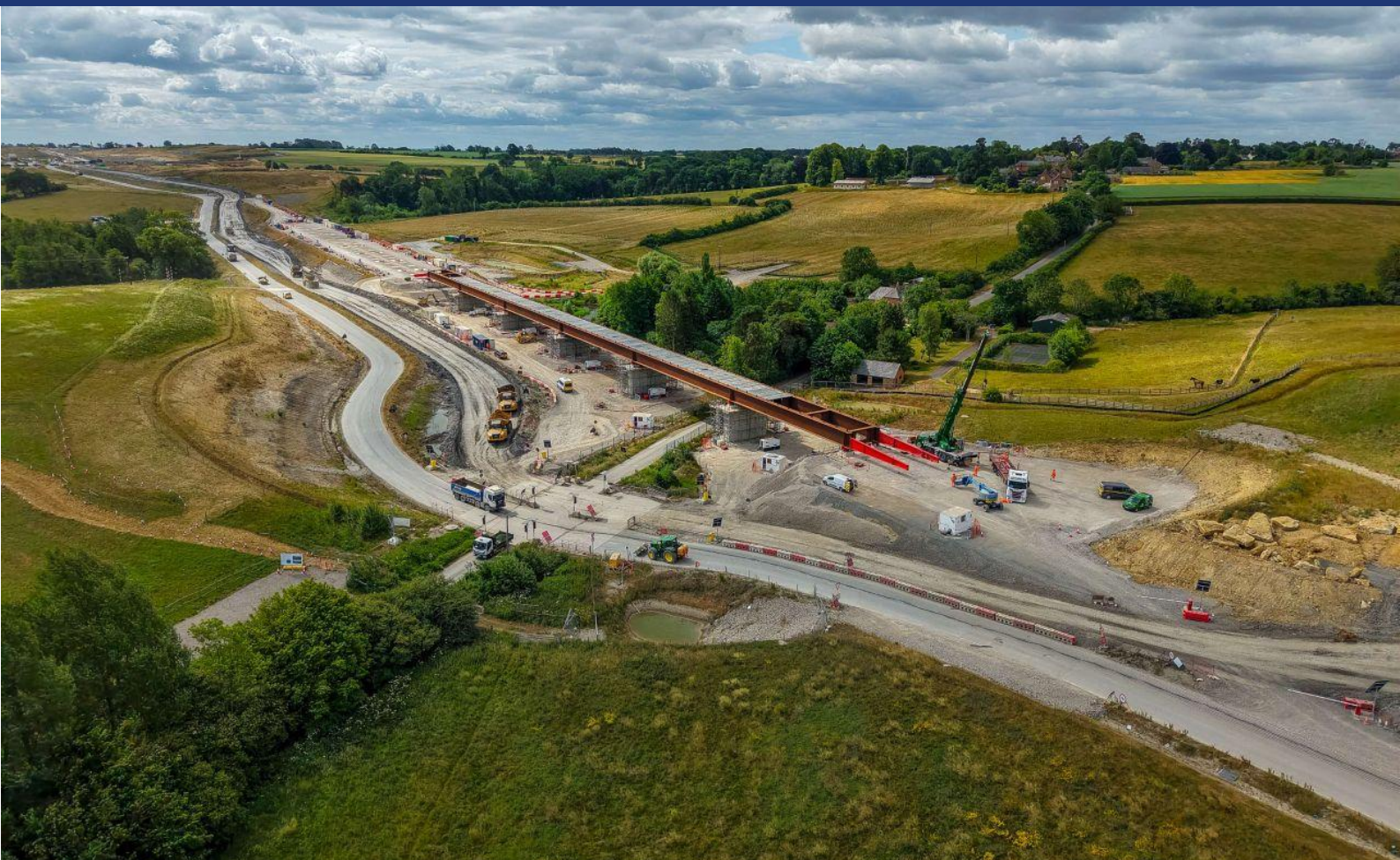
An aerial view of the Lower Thorpe viaduct deck installed in its final position
