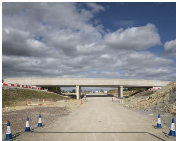
Kineton Road bridge will carry traffic over the HS2 railway line
