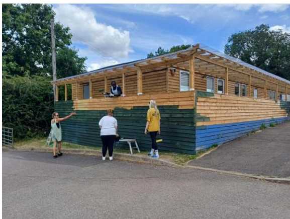
New and old wood was painted to preserve the new decking area at Woodford Halse food larder
