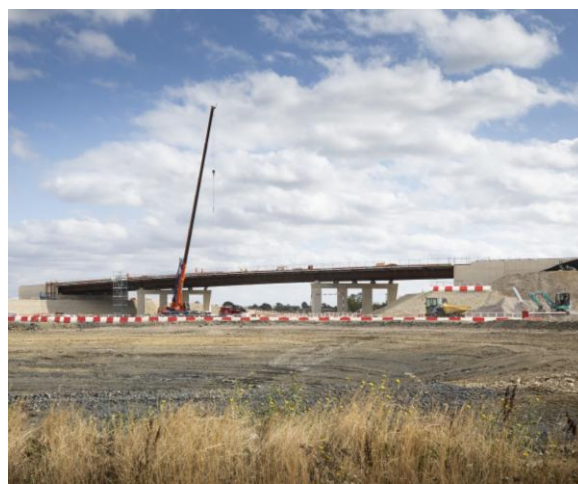
Cranes lift concrete deck slabs into place on the A423 road bridge near Southam
