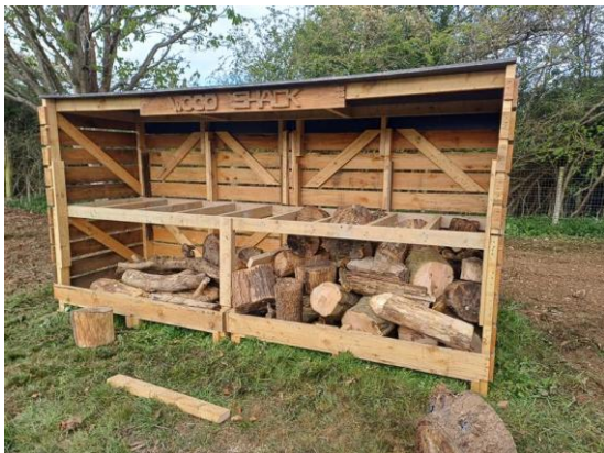
Our carpenters made this woodshed from recycled pallets to store wood for campfires
