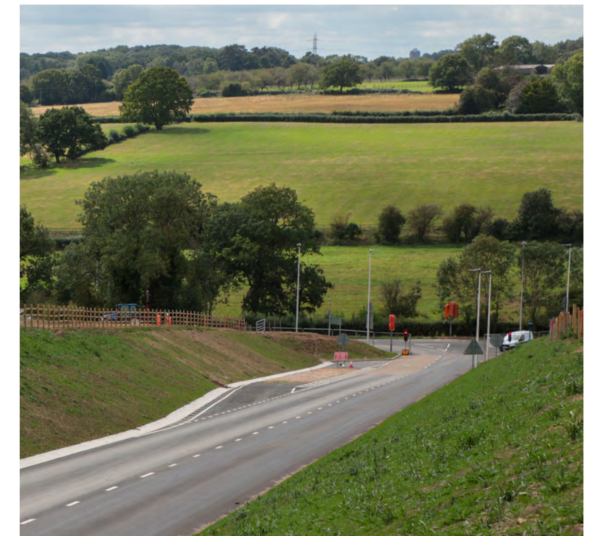
Temporary access road
