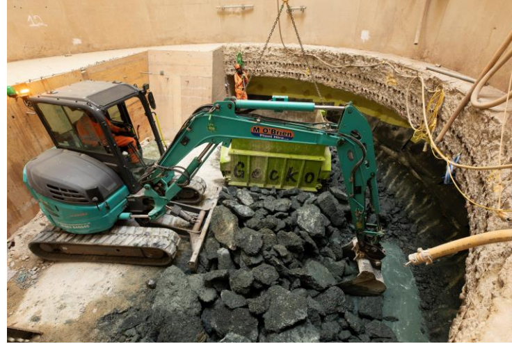
Excavation works bottom of satellite shaft
