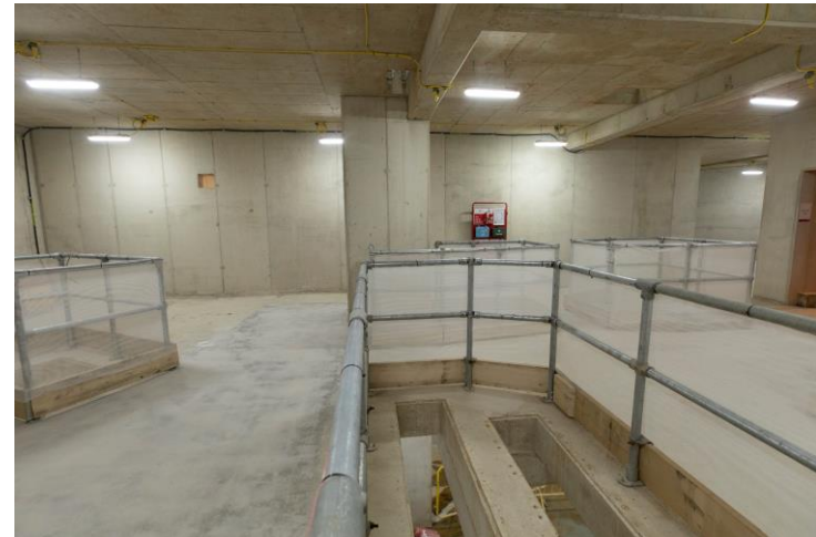
Walls, columns and slabs below ground in main shaft
