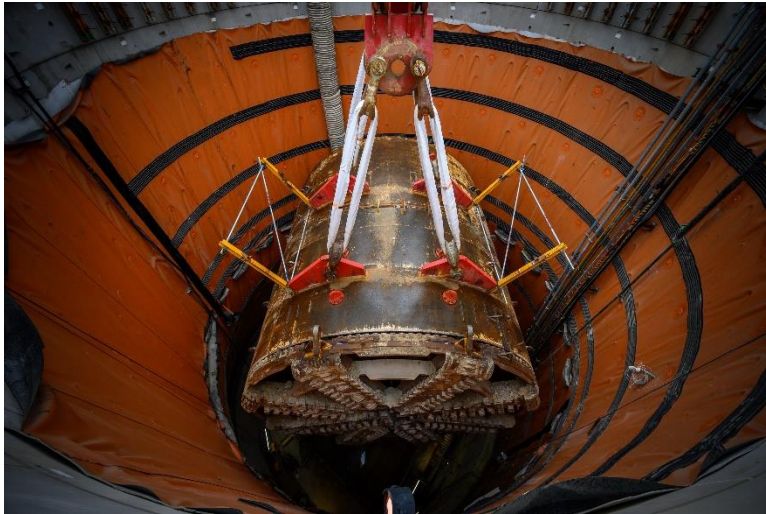
TBM Emily being removed from the Green Park Way Vent shaft site
