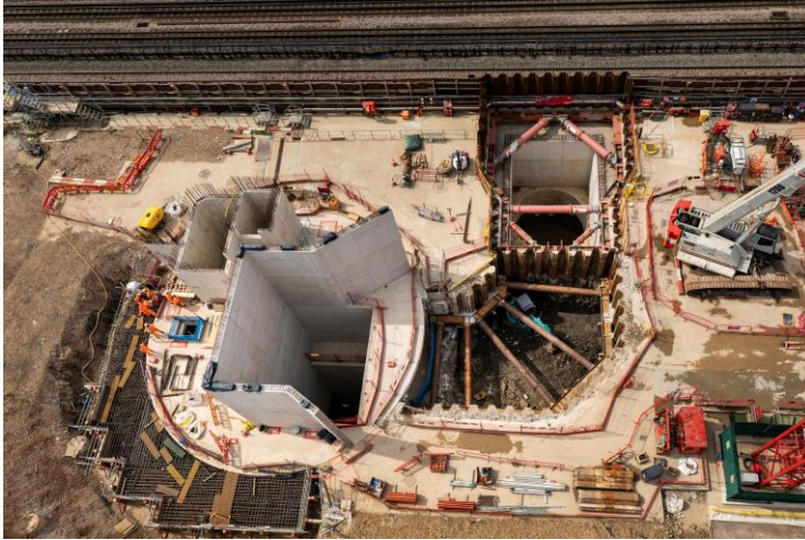
Aerial view of eastern end of the Mandeville Road site
