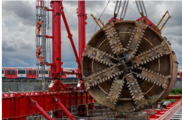
TBM Emily being removed from the Green Park Way Vent shaft site
