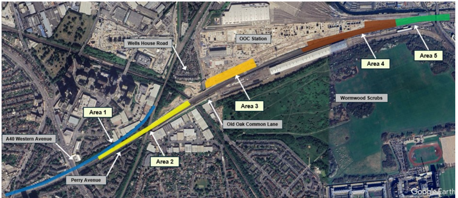
Overhead view of worksites
