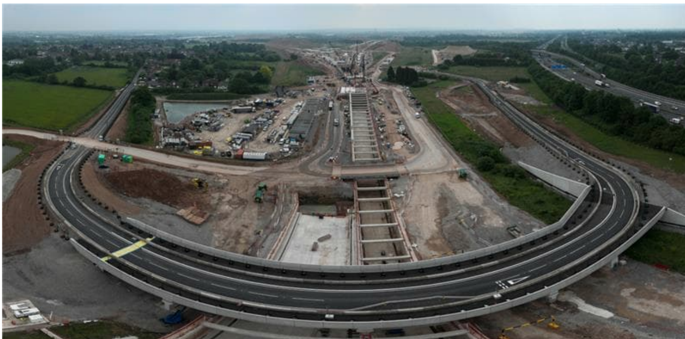
Works on the Attleboro Lane Overbridge
