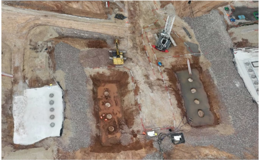
Church Lane works
