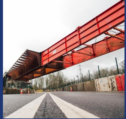
Small Dean viaduct across the A413 during the deck slide
