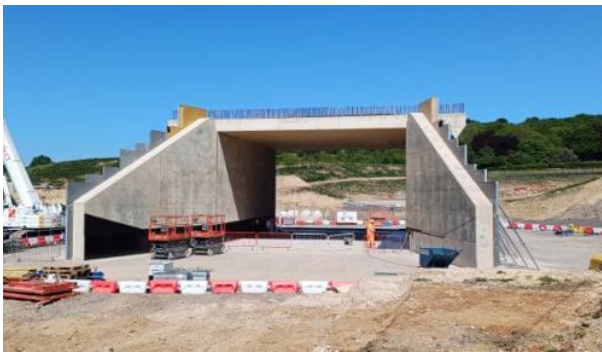
Rocky Lane underbridge under construction, wing walls concreted
