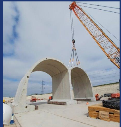
First segments being installed at Wendover green tunnel
