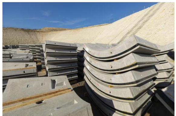
Pre-cast segments at the Grove Farm culvert
