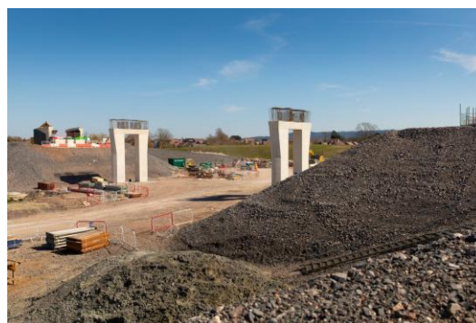
Above - SMA/9 overbridge piers under construction
