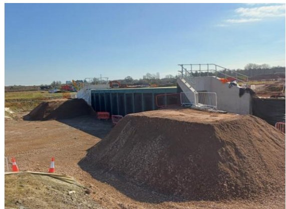
Above - Hartwell culverts prepared for
