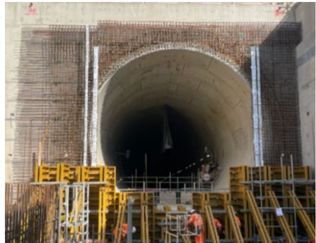
Constructing the reinforced concrete structures within the former launch chamber and portal
