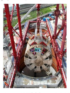
This process will be repeated for TBM Emily and Anne. The front of the TBM (the cutterhead shield) will be separated from the tunnelling support structures (the body of the TBM). The cutterhead shield will be cut into sections so that it can be lifted out of the shaft using a large crane.
