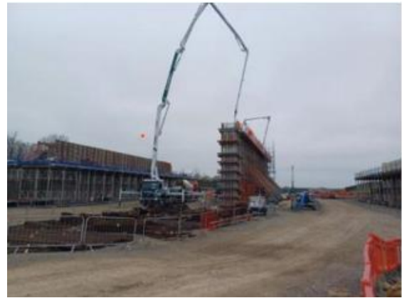
The image above shows the piers being poured at School Hill overbridge
