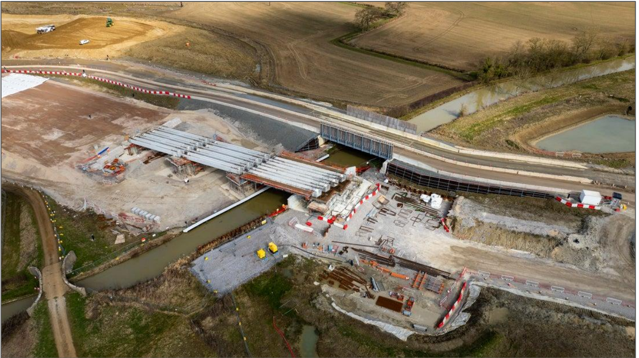
All the deck beams for the Oxford Canal viaduct, near Wormleighton have been installed.
