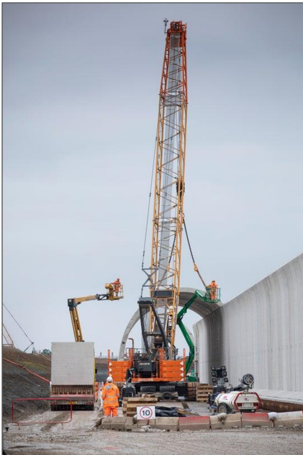
Tunnel segments are installed by crane
