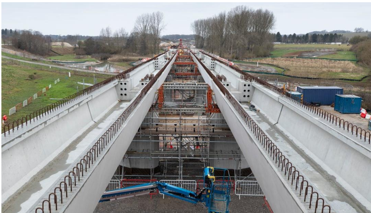
View of the beams installed on the Edgcote viaduct, near Chipping Warden
