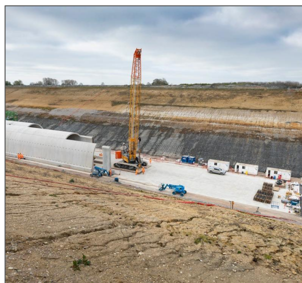
In the Greatworth green tunnel layers of geology can be seen in the excavation.
