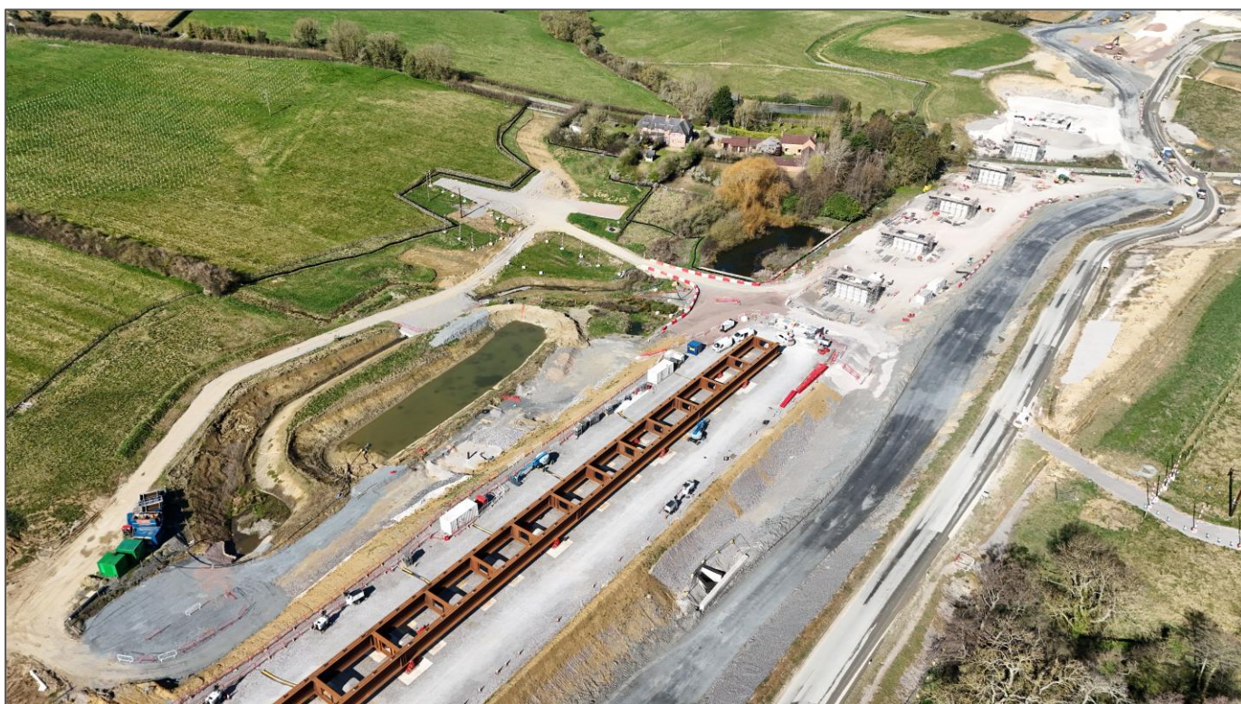
The metal frame for the Lower Thorpe viaduct is being prepared to launch over the viaduct piers
