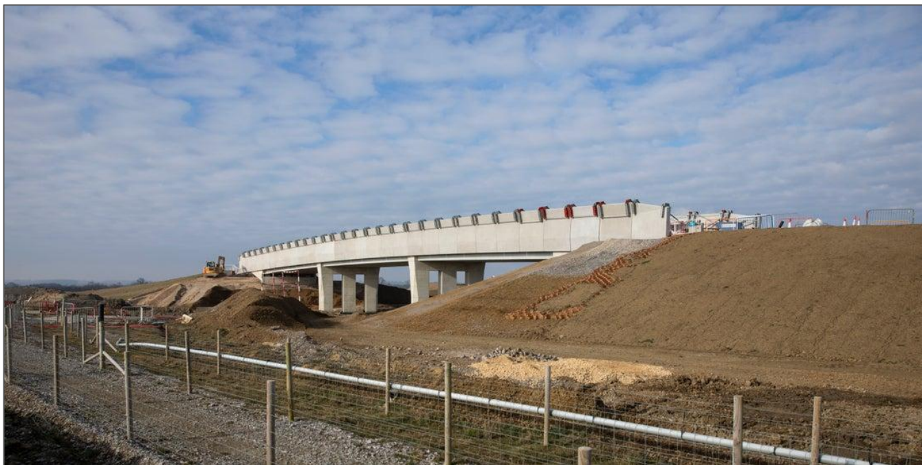
Parapets have been installed at Claydon Road overbridge, Lower Boddington
